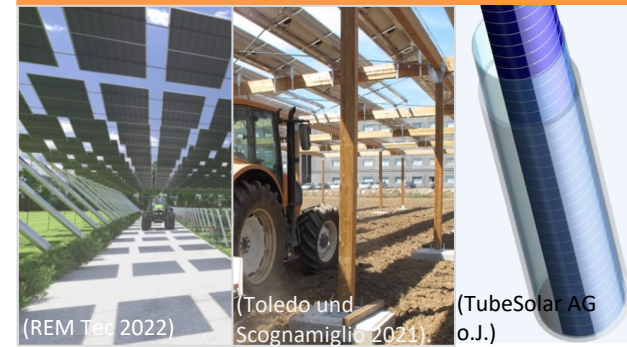
Figure 3: a) rope construction, b) wood construction, c) tube panels.
