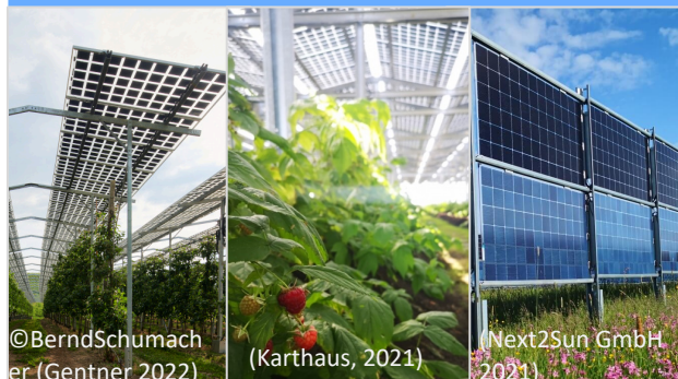
Figure 2: a) high elevated, b) low elevated, c) vertical agrivoltaic system.
